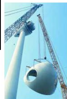
The spinner completes the form of the nacelle.
