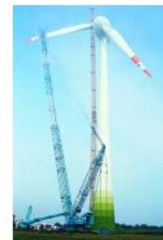
The second rotor blade is in place.
