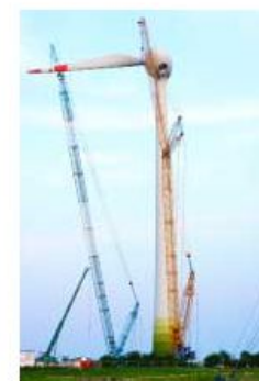
The first rotor blade is lifted.
