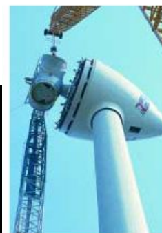
The hub being lifted by both cranes.
