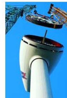
The disc rotor follows assembly of the stator.
