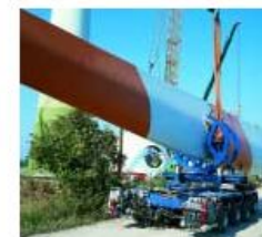
A rotor blade before being mounted on site.
